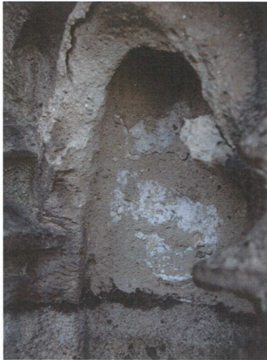
Fig. 12. Salt damage on Weibern tuff due to \text{Na}_2\text{SO}_4 on a pinnacle on St. John's cathedral 's-Hertogenbosch (picture R.P.J. van Hees, 2002).
