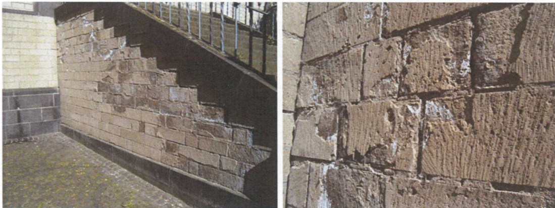
Fig. 13. Salt damage of Weibern tuff, St. Maria im Kapitol, Cologne (pictures T.G. Nijland, 2009).
