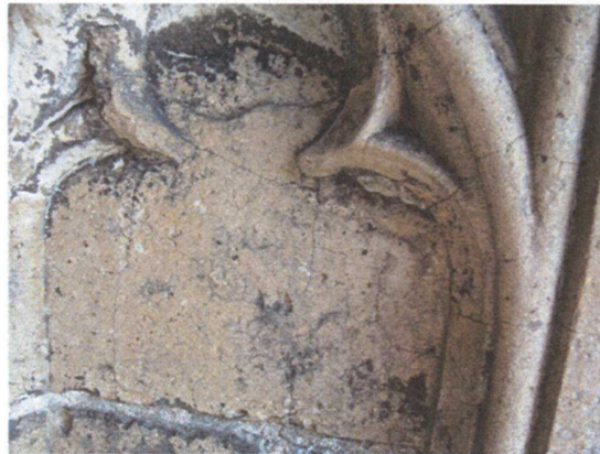
Fig. 6 Example of the formation of a hard, dark crust with craquelé on Weibern tuff at a pinnacle of St. John's cathedral, 's-Hertogenbosch (picture T.G. Nijland, 2006).
