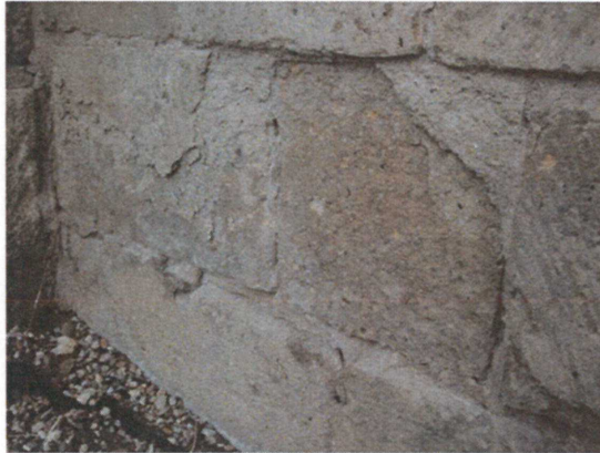
Fig. 2. Exfoliation of Weibern tuff directly above the ground level on the Grote Kerk, Oosterbeek (picture R.P.J. van Hees, 2002).
