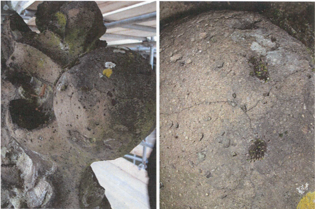
Fig. 7. Example of the formation of a hard, dark crust with craquelé on Weibern tuff ornaments on the rampant arches of St. John's cathedral, 's-Hertogenbosch (pictures R.P.J. van Hees, 2003).
