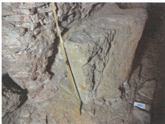
Fig. 3. Block of Römer tuff in the Roman thermae in Heerlen (picture T.G. Nijland, 2016).
