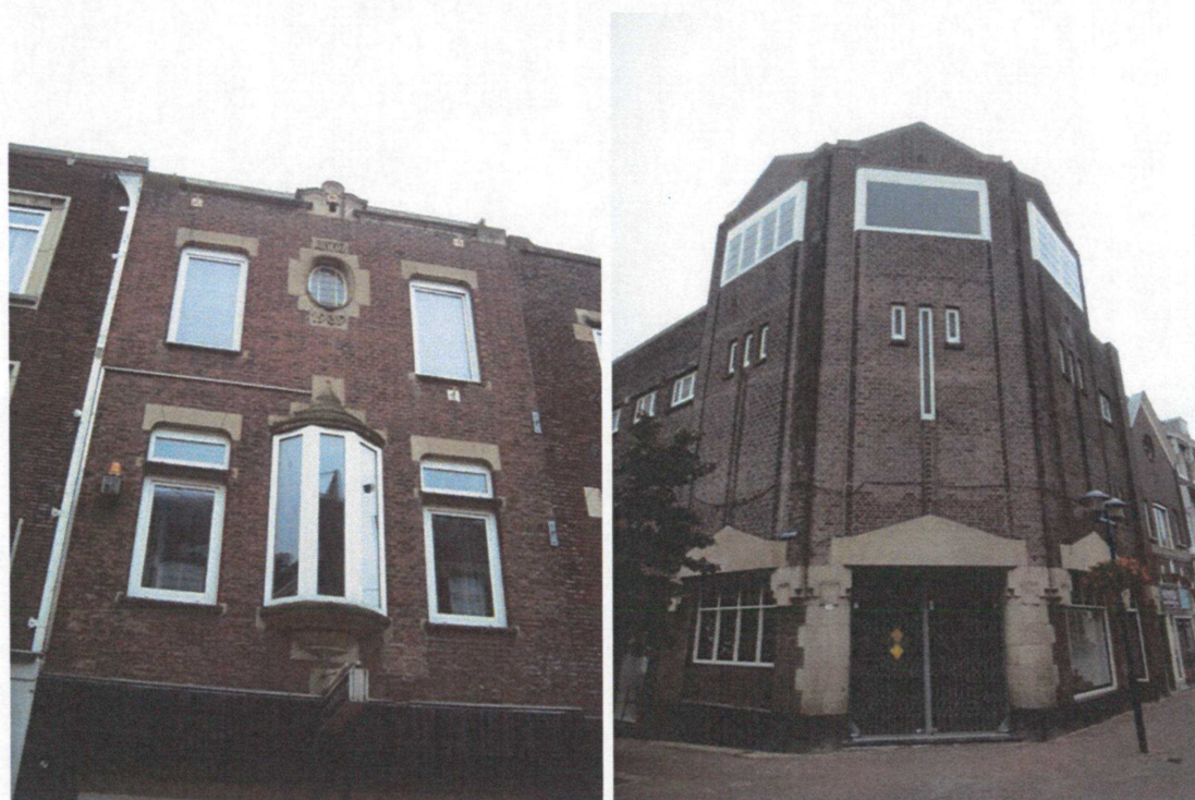
Fig. 15. Ettringen tuff building parts in red clay brick masonry. Left a residential building at Hogehuisstraat 13, Eindhoven, built 1939, right Hoogstraat 99, Schiedam (pictures T.G. Nijland, 2008 and 2014).
