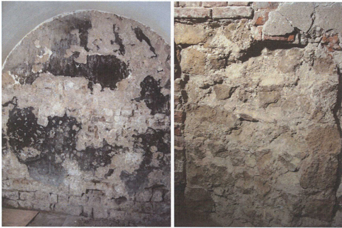
Fig. 1. Remains of the Roman castellum wall in a cellar below a late Medieval house at the Dom square, Utrecht. The left picture shows part of the wall, of which the lower part is original Roman masonry (ca. 210 AD), whilst the upper part was rebuilt in pre-Medieval times. The right picture shows a cross-section of the wall in another part of the cellar (pictures T.G. Nijland, 2009 (before the transformation)).
