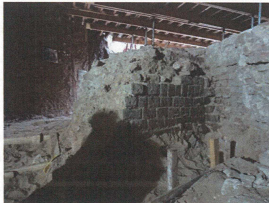
Fig. 2. Remains of Roman formwork in Römer tuff, excavation below the Stratemakerstoren at the foot of the Valkhof, Nijmegen (picture T.G. Nijland, 2017).
