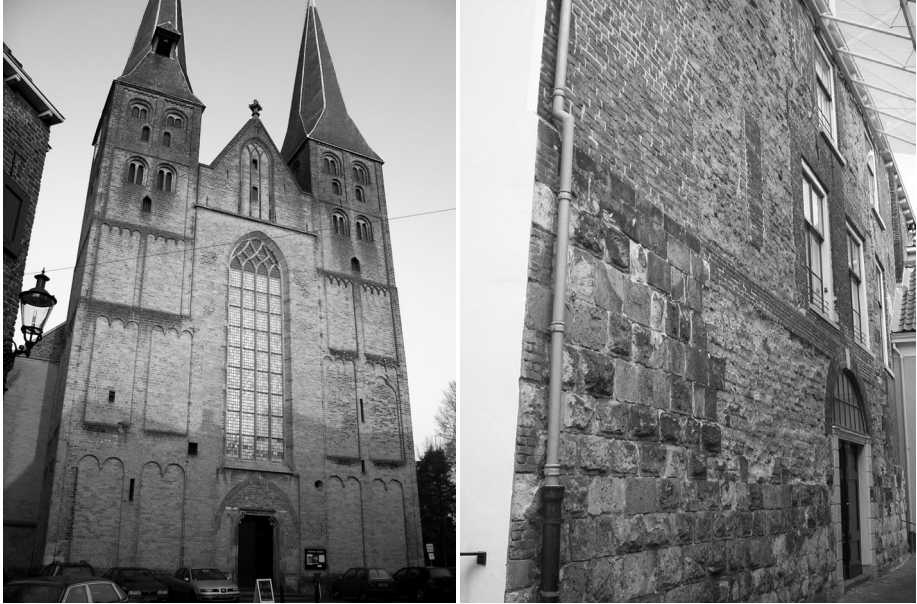
Figure 2. Römer tuff in the staple town Deventer, left the Bergkerk (c. 1200); right the Deanery, the oldest surviving stone house in the Netherlands
