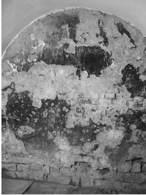
Figure 1. Remains of the Roman castellum wall in a cellar at the Dom square, Utrecht. The lower part is original Roman masonry (ca. 210 AD), the upper part was rebuilt in pre-Medieval times.
