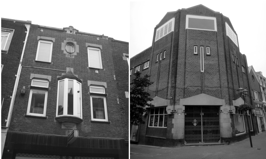
Figure 8. Ettringen tuff building parts in red clay brick masonry. Left a residential building at Hogehuisstraat 13, Eindhoven, built 1939, right Hoogstraat 99, Schiedam.
