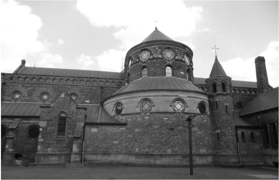
Figure 6. Ettringen tuff on the 1930's St. Jacques the Greatest church, Enschede, by architects H.W. Valk and J.H. Sluijmer.
