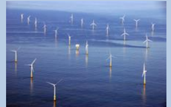
Figure 1. Off-shore wind farm
