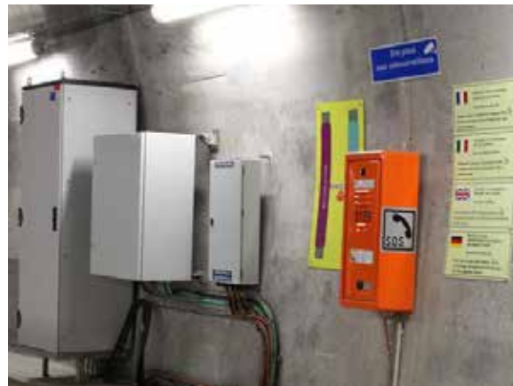
Illustration 17b - Tunnel A 89 (France)
