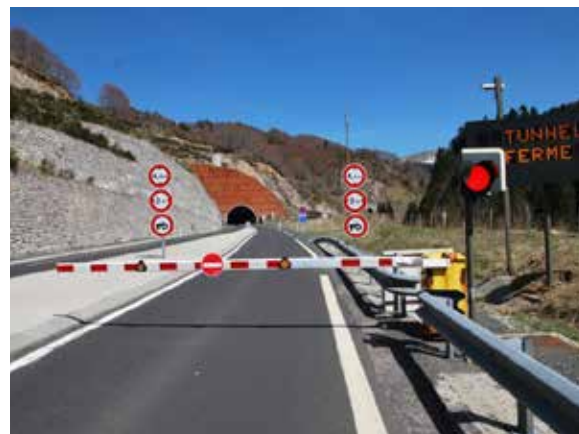
Illustration 9b - Lioran tunnel (France)
