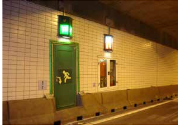
Illustration 15b - Noord tunnel (The Netherlands)
