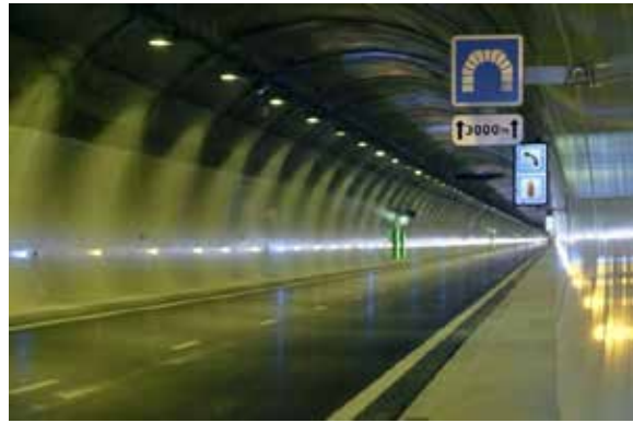
Illustration 6b - Violay tunnel A 89 (France)
