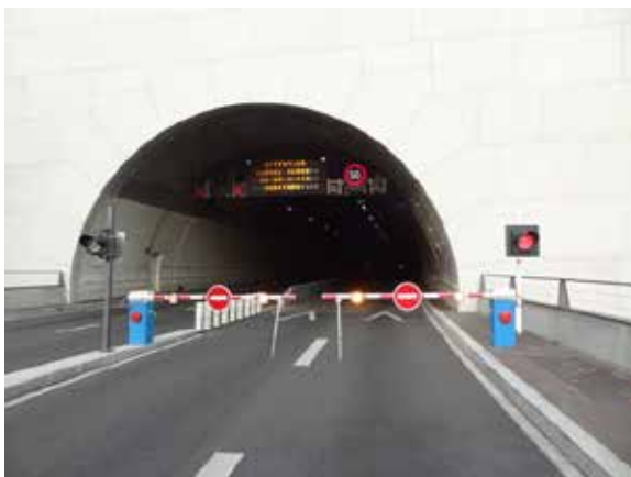
Illustration 9a - Croix Rousse Tunnel – Lyon (France)
