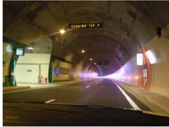
Illustration 8b - La Bussière tunnel A 89 (France)
