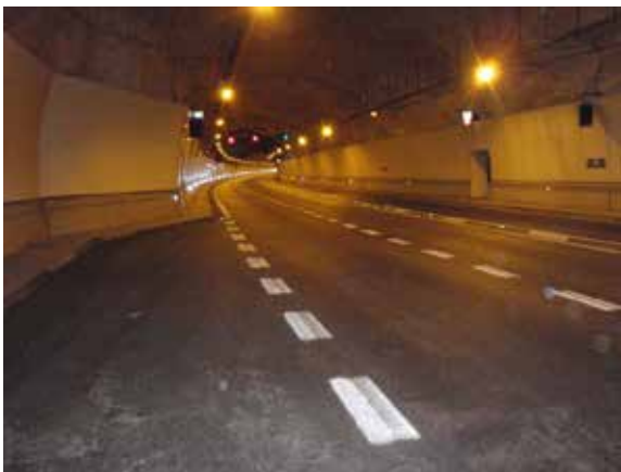
Illustration 11a - Bracons tunnel (Spain)
