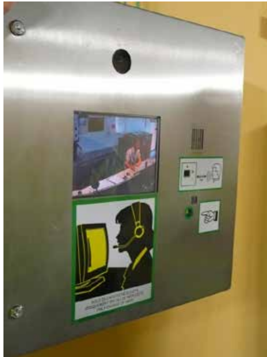
Illustration 16 - Example of videophones, Mont Blanc tunnel (France – Italie)
