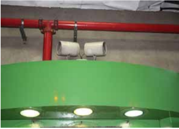
Illustration 15a - Cadi tunnel (Spain)
