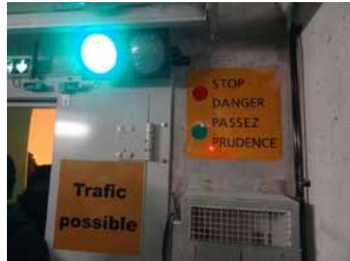
Illustration 18b - Talant tunnel (France)
