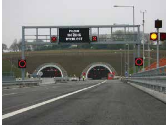
Illustration 7b - Klimkovic tunnel (Czech Republic)
