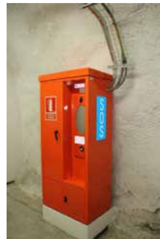
Illustration 12b - Cadi tunnel (Spain)
