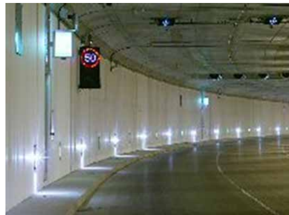
Illustration 11b - Tunnel in Switzerland
