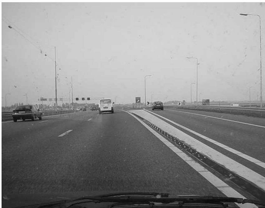
Figure 8 Picture of the led-light bar implemented on the A9 motorway in the Netherlands °
