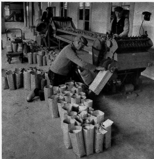
MECHANIZATION: BULB-COUNTING MACHINE (Courtesy of Zonneveld & Philippo N.V.)
