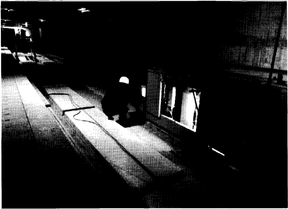
Figure 51 The Autonomous drilling robot at work in the railway station at Schiphol.
