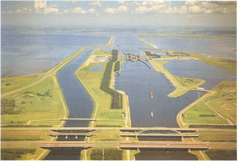
Bath Discharge canal and Scheldt-Rhine canal. In the centre the Kreekrak Locks
