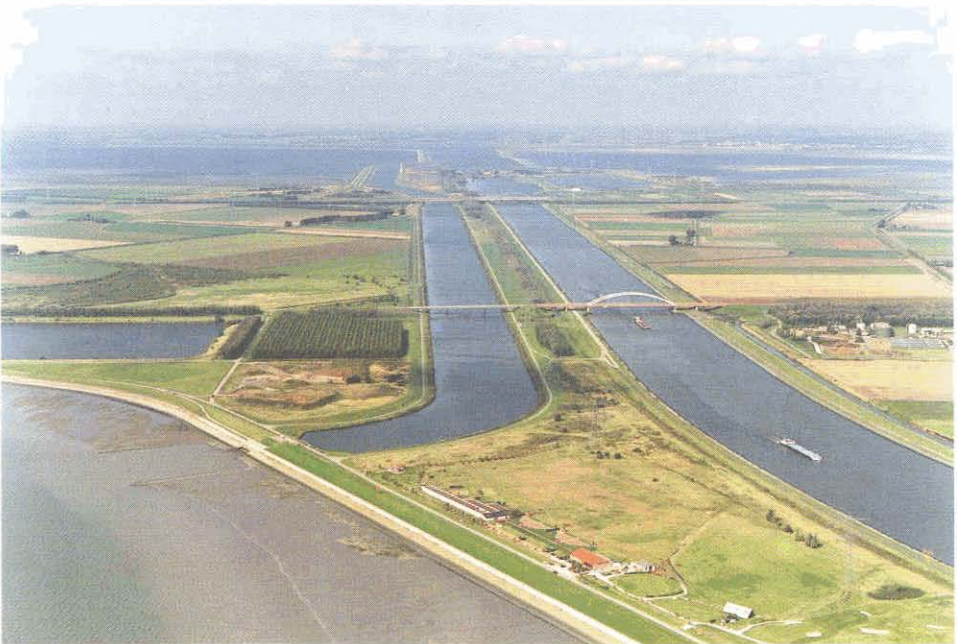
Bath Discharge canal and sluices
