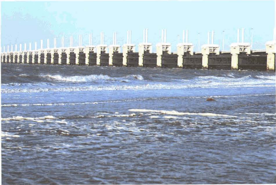
Storm surge barrier Eastern Scheldt
