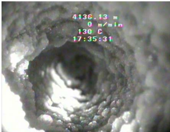
Figure 10. NaCl scale in the perforated zone (well F16-A1).
