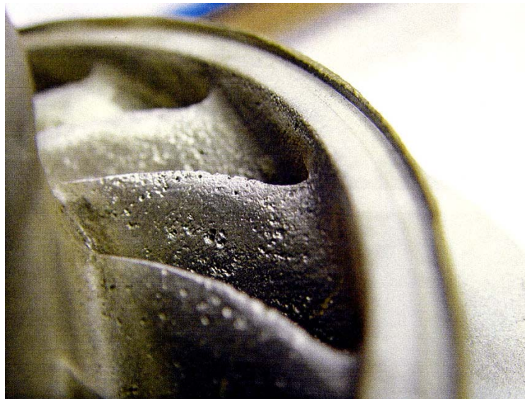
Figure 21. Corrosion and pitting noted at the impeller.
