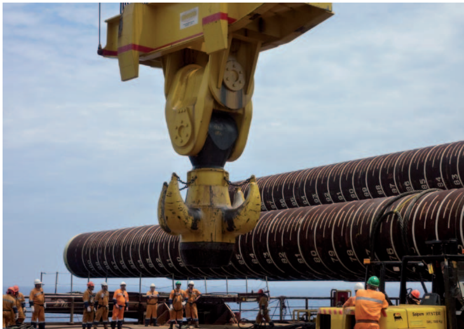
Preparations are taken to up-end the piles
