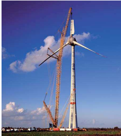
Figure 2.6: The Enercon E-126 prototype features a divided blade (Image: Enercon)
