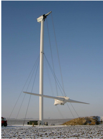
Figure 2.7: The Vergnet 1 MW turbine does not need a large separate crane for installation (Image: Vergnet)
