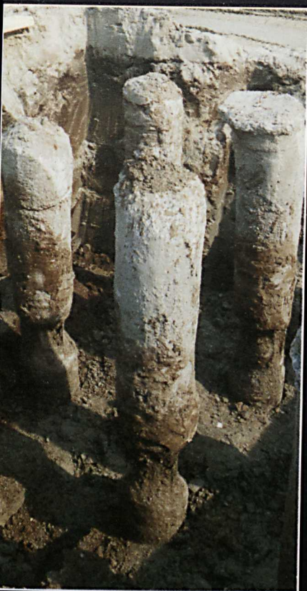
sonic integrity testing
