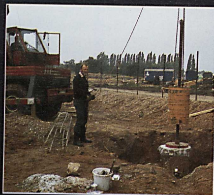
dynamic load testing
