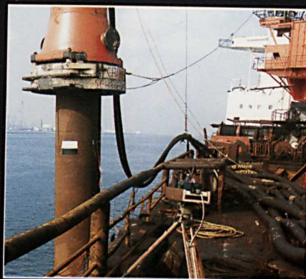
pile and hammer monitoring
