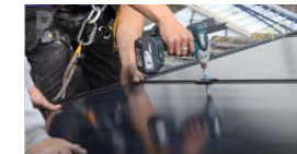
4. Vastzetten panelen
