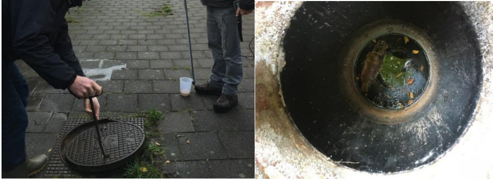
Figure S3.1.3 Example of a manhole of the groundwater drainage system (the dead fish indicates the possible back flow from the ditch to the drain manhole)
