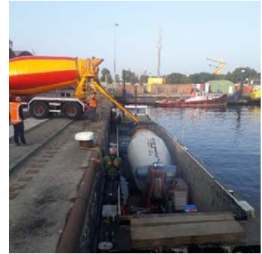
Figuur 9: Beton over water
