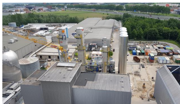
The ECN.TNO designed 100 kton/y CO 2 capture installation at the waste to energy plant of AVR.
