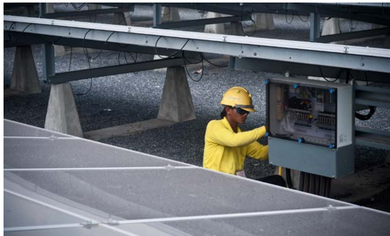
Lopburi solar power plant, central Thailand. (Photo credit: Asian Development Bank)
