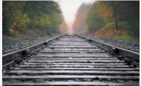
What about automation in rail transport? (Idfi, 2015)
