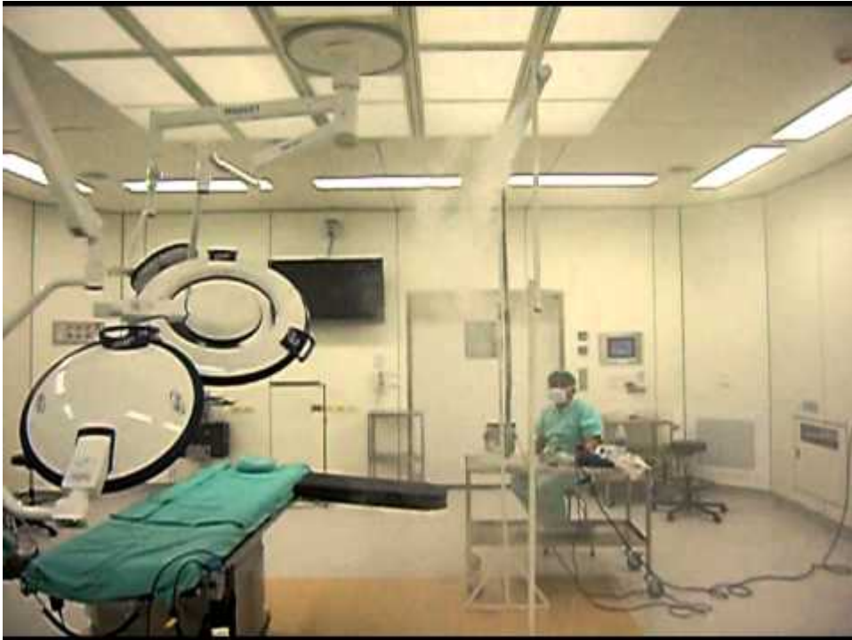
Workshop Hospital Ventilation
