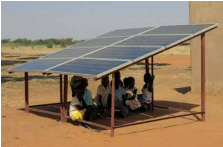
Figure 22. Solar power panels in a community.
