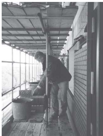
Figure 2. Raised bricklaying with consoles.
