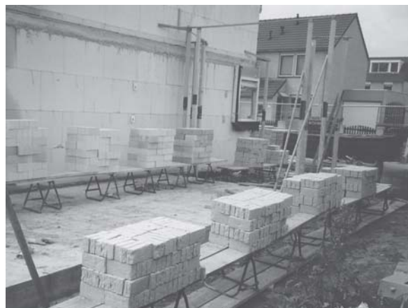
Figure 1. Raised bricklaying with stools.
