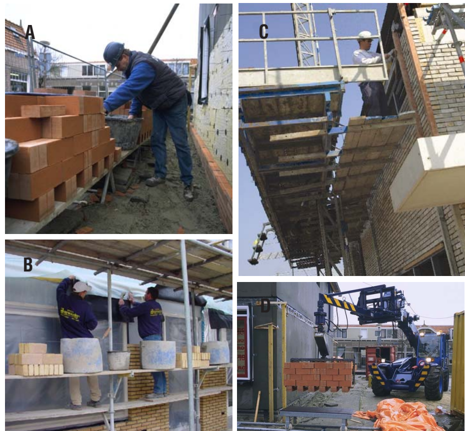
Figure 1. Examples illustrating the four types of ergonomic measures implemented in the companies and the teams of bricklayers and bricklayers' assistants: use of a trestle (A), a bricklaying scaffold (B), a mast-climbing work platform (C), and a crane (D).
