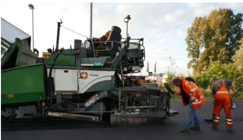
Figure 2: Laying a test road section
