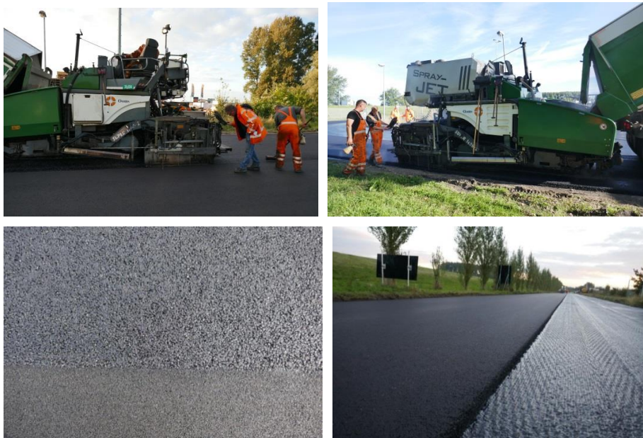
Figure 3: Road sections for field testing
