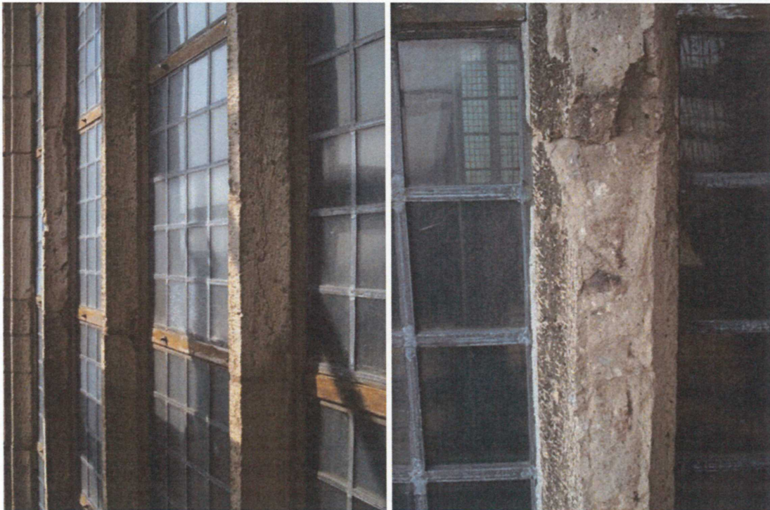
Fig. 2. Typical longitudinal cracking (left) and final damage in mullions of Weibern tuff at the nave of St. Peter's church in Leiden, The Netherlands (pictures T.G. Nijland, 2005).
