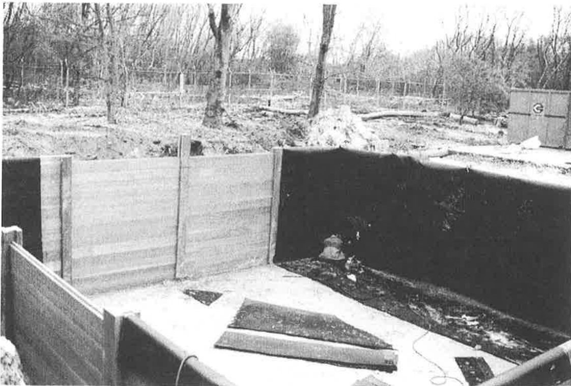
Figure 3.8 The inside of the box is covered with a watertight plastic lining in order to prevent pollution from the outside (for example ground water) entering the box.
