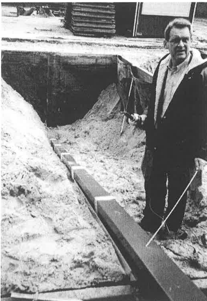
Figure 3.12 Installation of a square PVC tube running from the surface of one side to the bottom of the other side of the box, facilitating measurements of EM transmissions into the ground.
