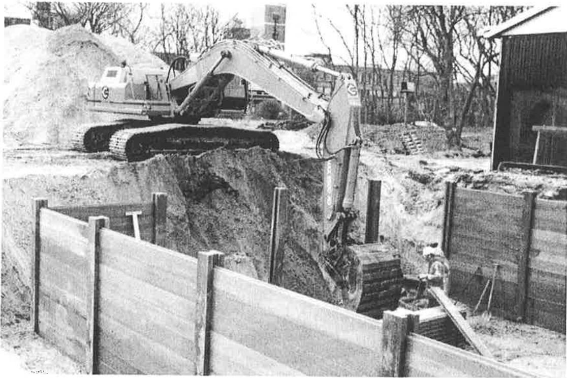
Figure 3.6 Last part of the digging phase. The wooden box is almost finished.
