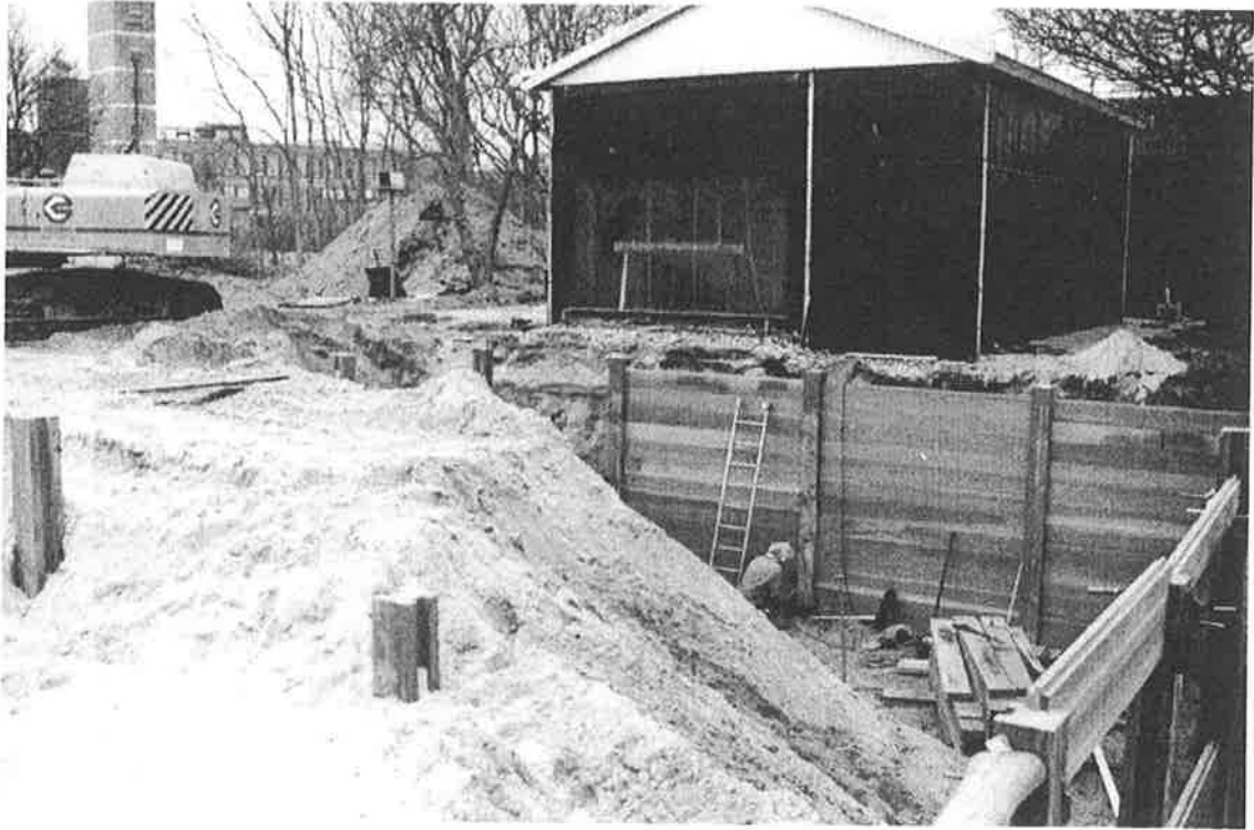
Figure 3.5 While the walls of the box were being constructed, the soil at the location was removed simultaneously.
