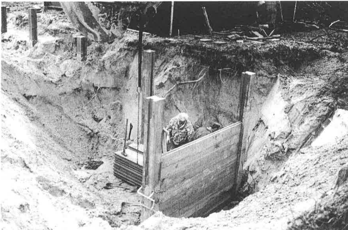
Figure 3.4 Construction of the walls of the box using wooden beams. The wood that was used to construct the box was tropical hardwood from Central Africa.
