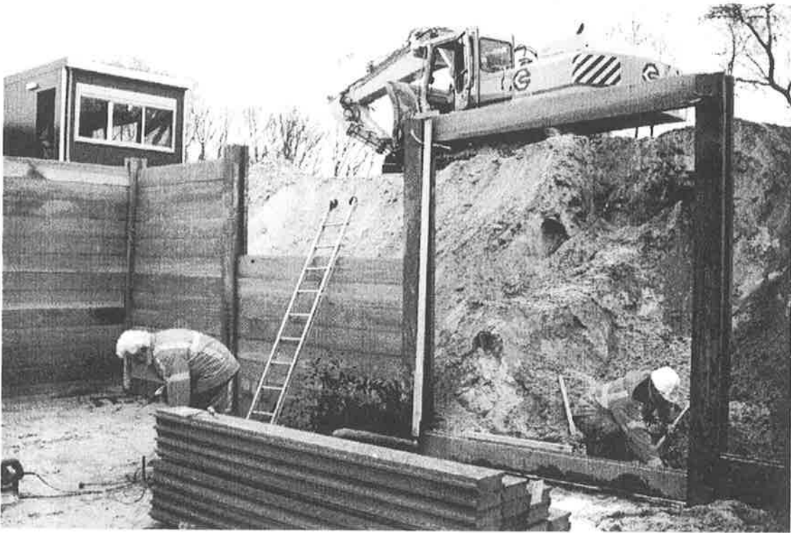
Figure 3.7 Closing of the wooden box.
