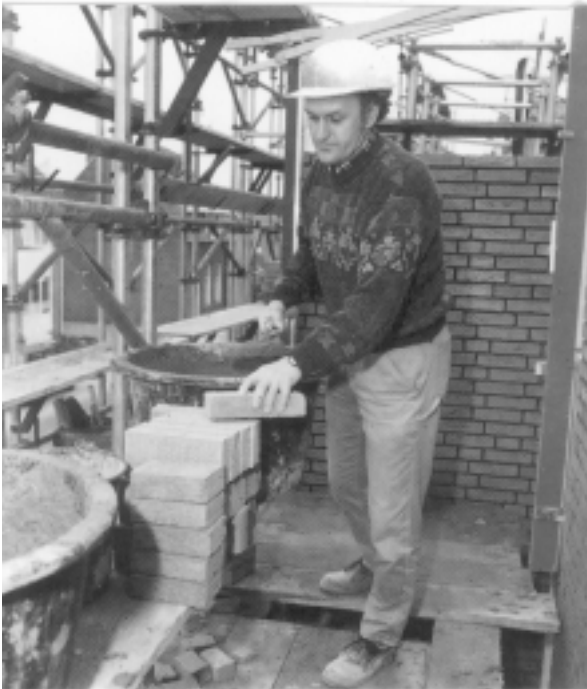
Figure 2. Bricklaying with a split floor scaffolding with bricks and mortar 50 cm raised.
