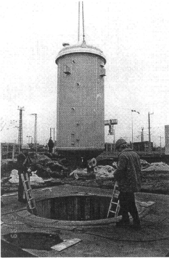
Fig. 2. Installation of a reactor (length 2,5 m, diameter 1,4m)
