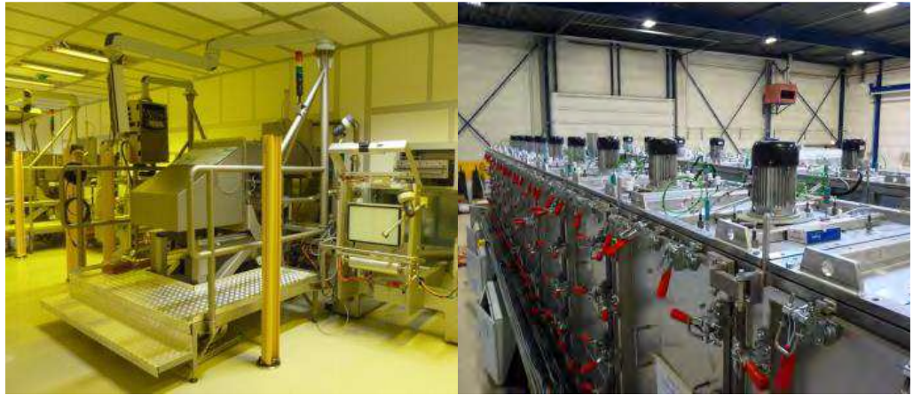
The novel Solliance roll-to-roll line constructed by VDL-ETG for PSC processing, viewed from the coating site in the clean room of the Solliance building at HTC21.
