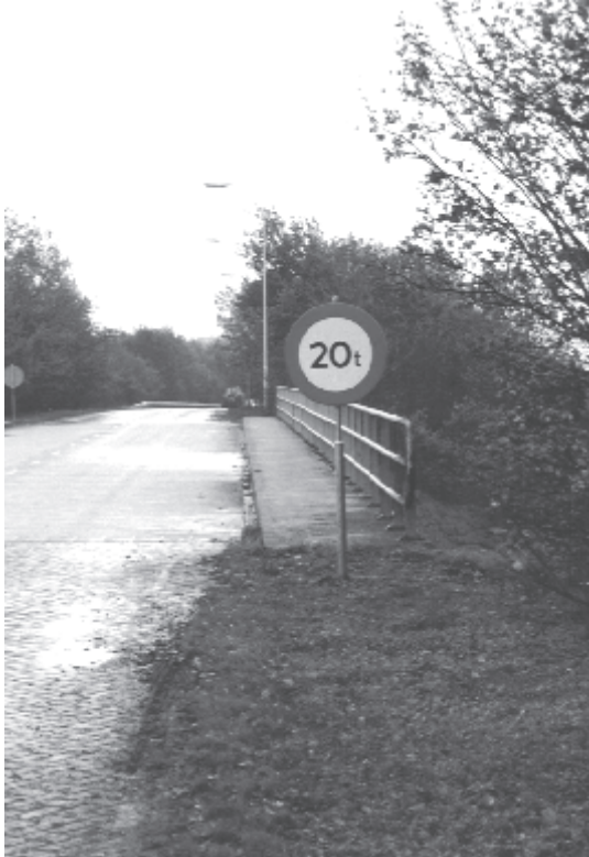
Figure 1. Load limitation to 20 tonsting on a viaduct due to a reduction of the load-bearing capacity from ASR
