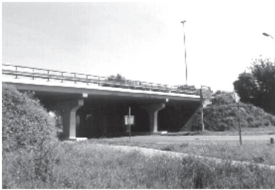
Fig. 1. Overview of viaduct Wolput.
