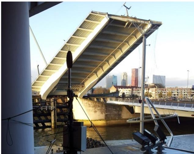
Figure III: Open bascule bridge, northward view, showing main bearing girders and bridge deck with stiffening profiles.
