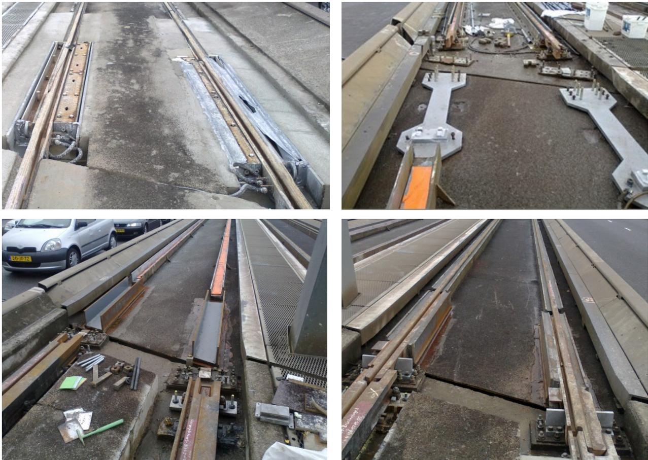
Figure XI: Noise control measures during track renovation. Top left: Diagonal rail joint based in concrete; top right: added mass and stiffness at joint 4; Below : added stiffeners at joint 4, left without rails, right with rails and cork rubber embedding and seatings for bascule bridge rails.
