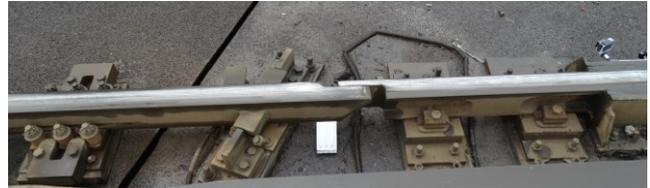
Figure V: Rail joint 4 with from left to right: suspension support, seating support, 2 clamp supports with railpads and far right, embedded rail. The rail on the left moves with the bascule bridge and 'lands' on the seating support which is on a concrete base..
