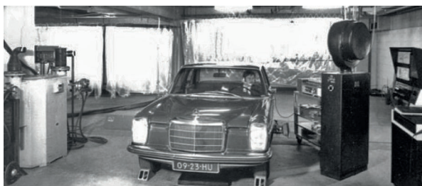
Chassis dynamometer TNO – Mobility, Delft 1970.
