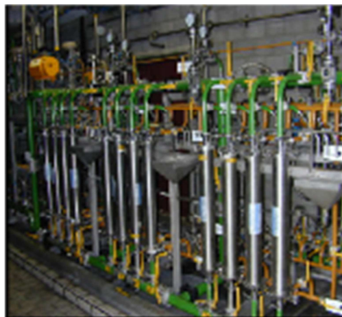
Example of modular separation technologies: modular membrane extraction (pertraction) process for waste water treatment implemented by TNO at Invisita, the Netherlands
