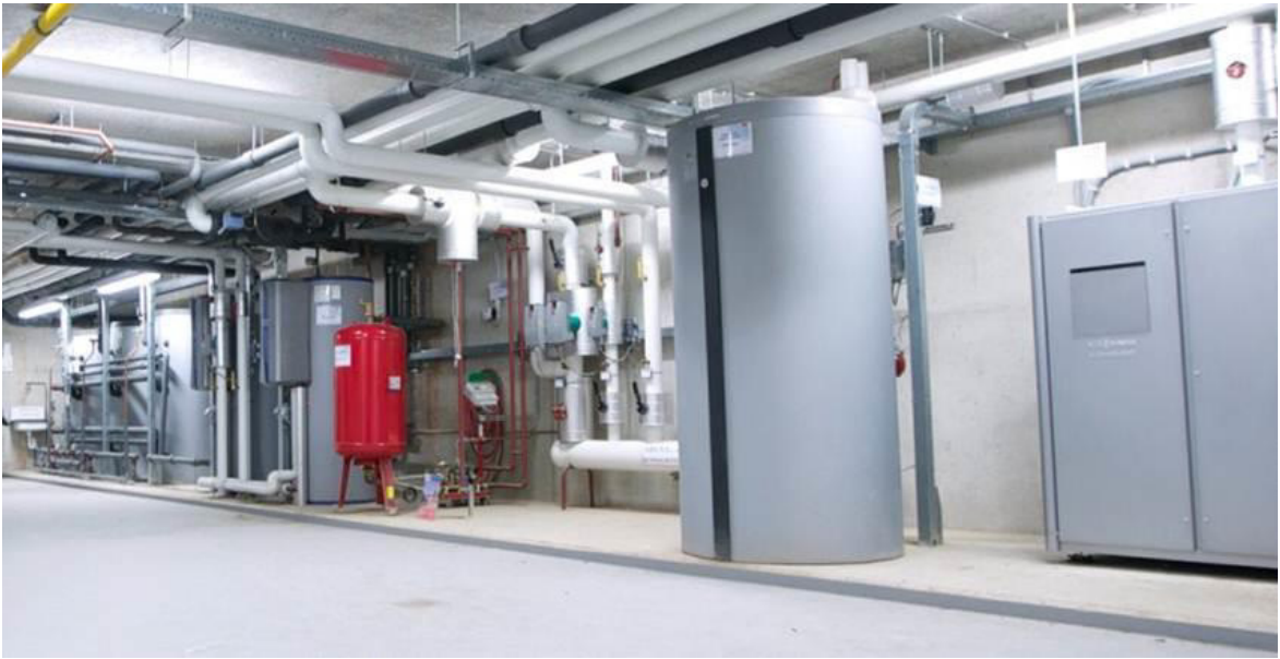
Fig. 4. The installation used for the field test with heat pump, buffer and plenum.
