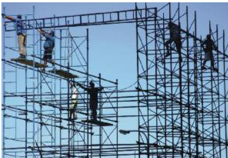
Dangerous construction site. Author: Peter Rimmer
