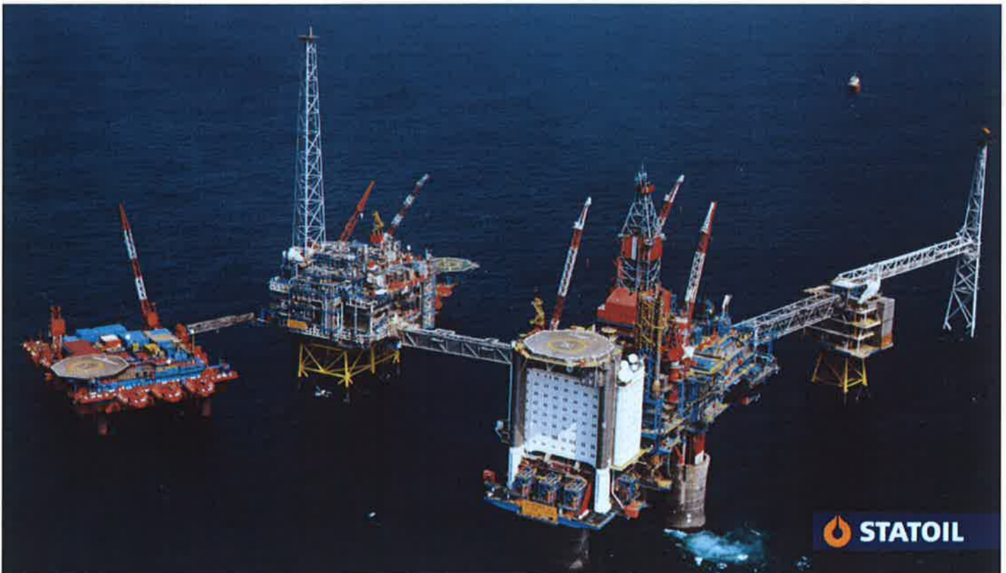
The Sleipner platform (Courtesy Statoil)
