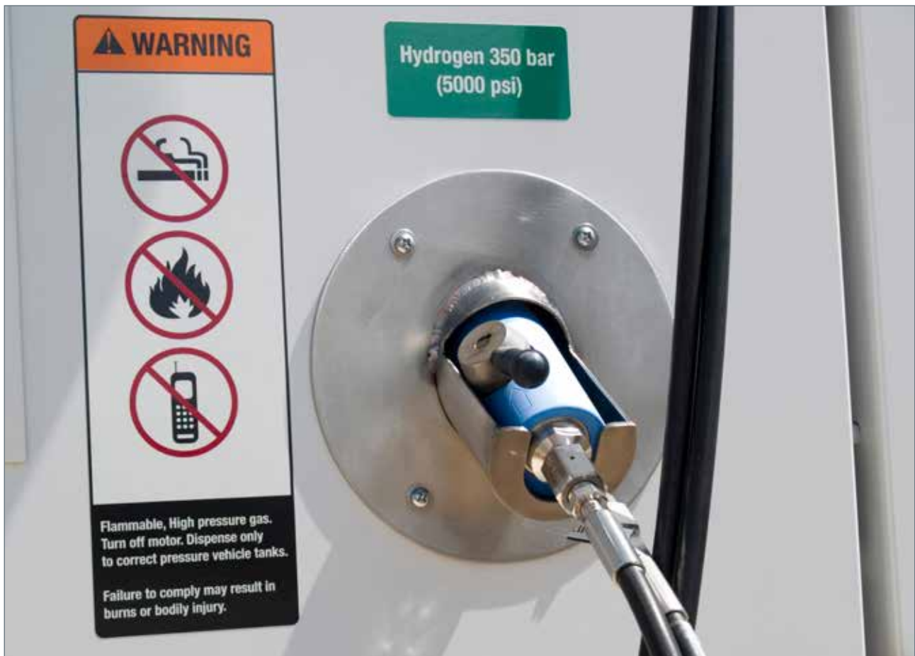
Figure 14. Hydrogen dispenser for vehicles.
