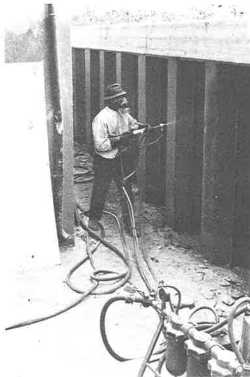
Fig. 15: The coating procedure of a bridge abutment at Hamm
