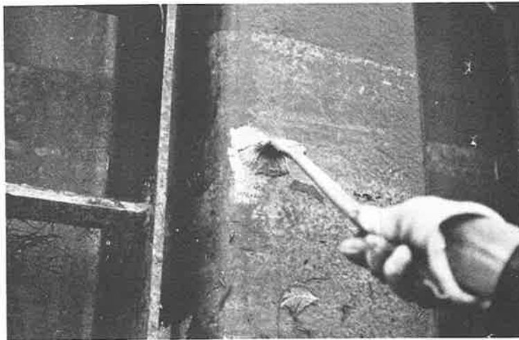
Fig. 13: Repair procedure of PUR-coated sheet piles at Bengersiel
