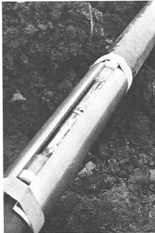
Fig. 17: Applying of a circumferential weld
