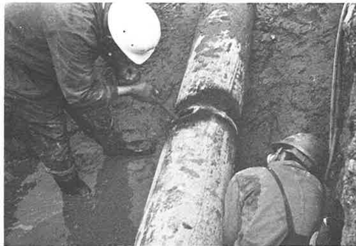
Fig. 21: Removing of damaged coatings
