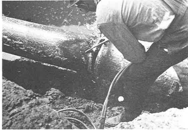
Fig. 20: Fire retarding PUR-coatings allow welding
