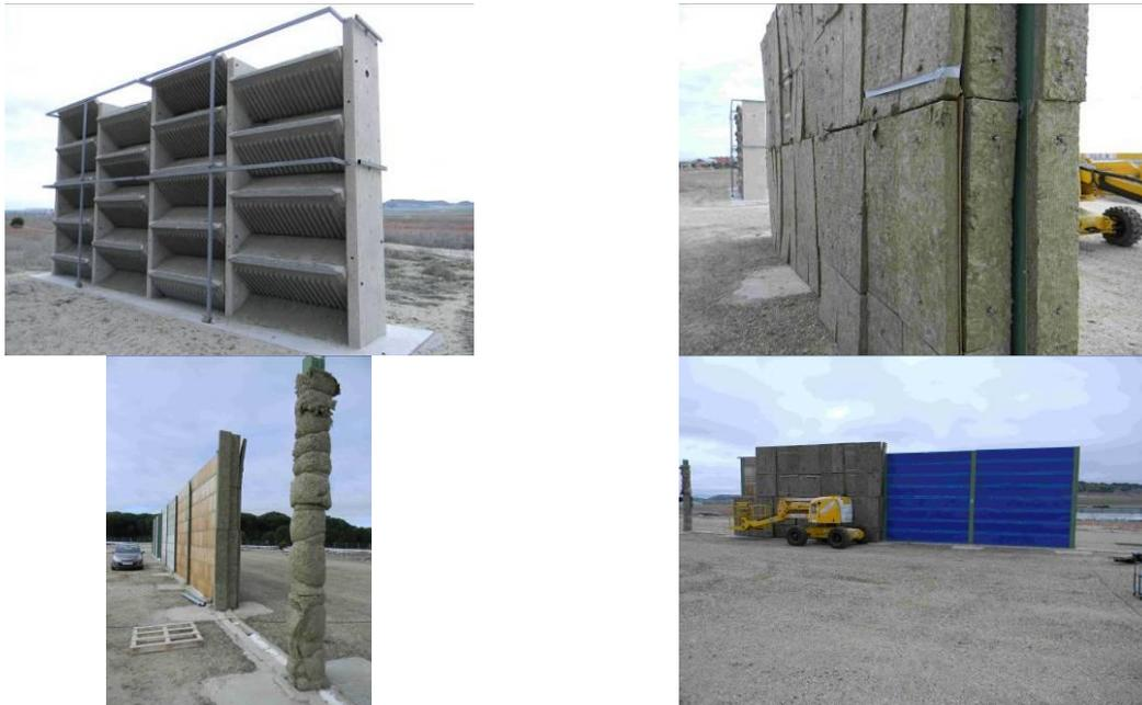
**Figure 43 - Metallic frame (upper left) and acoustic curtain installed. Metallic post covered with acoustically absorptive material (bottom left)**
