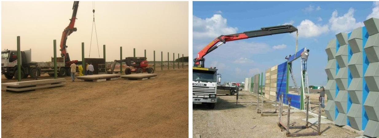
**Figure 35 - Metallic posts preinstalled before NRD assembly (left) and assembly of NRDs (right)**
