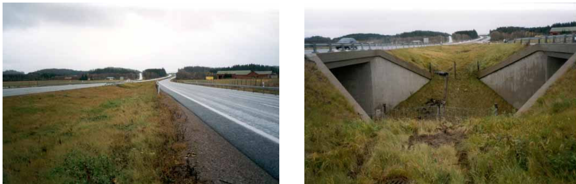
Figure 4.9. Hazardous underpass on motorway, notice too short safety barriers
