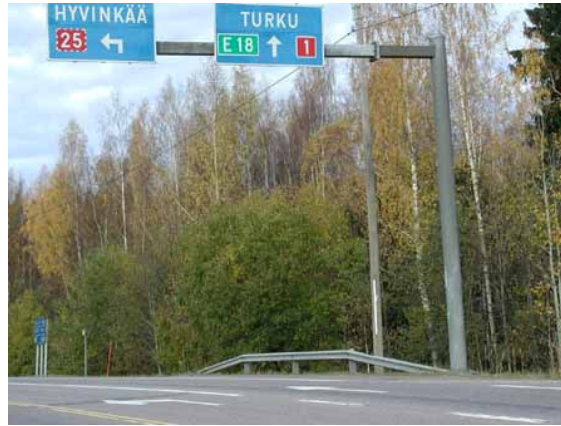
Figure 4.5. The culvert is protected with a short guardrail but the gantry pole and the old rigid lighting column are unprotected (Photo, HUT)
