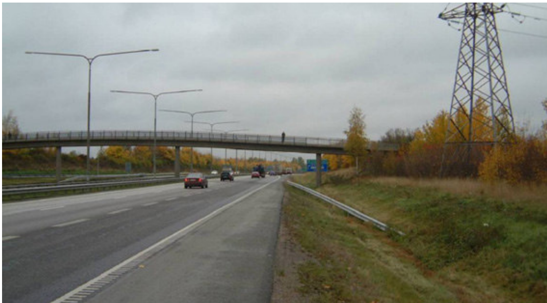
Figure I.2. Self Explaining Road with Forgiving Roadside
