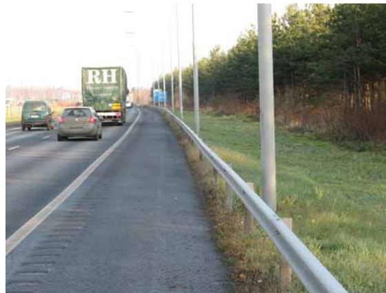
Figure 4.4. Rigid Lighting Columns protected with Guardrail
