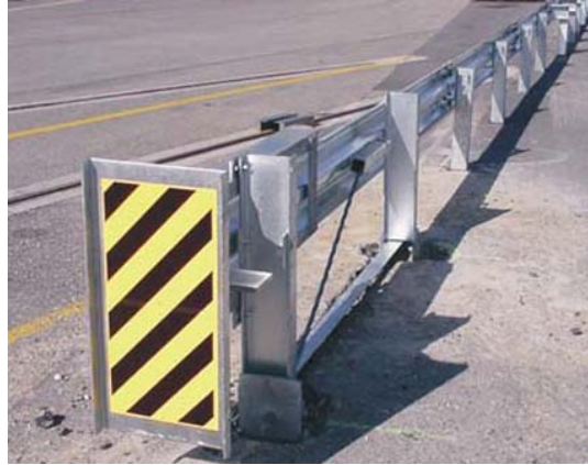
Figure 5.2. Safety Barrier Terminal
