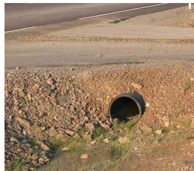
Figure 4.11. Examples of culverts in minor road junctions: traditionally the ends are vertical and the side slopes of the minor roads steep which makes them very hazardous objects in collisions (Photo, HUT)
