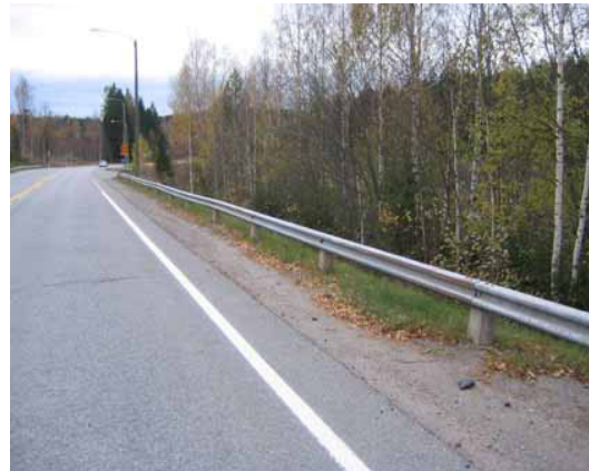
Figure 4.6. Examples of the distributed hazards. Left: unprotected rock cut very close to the carriageway. Right: untested guardrail with concrete posts and too low positioning (Photo, HUT)
