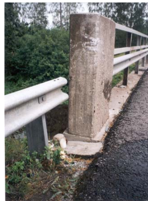
Figure 4.27. Left: good solution of transition structure, the guardrail is overlapped with the concrete barrier and fastened with steel bolt. (Photo, HUT) Right: poor solution of the transition from steel guardrail to the concrete pillar of the bridge parapet. (Photo, VALT)
