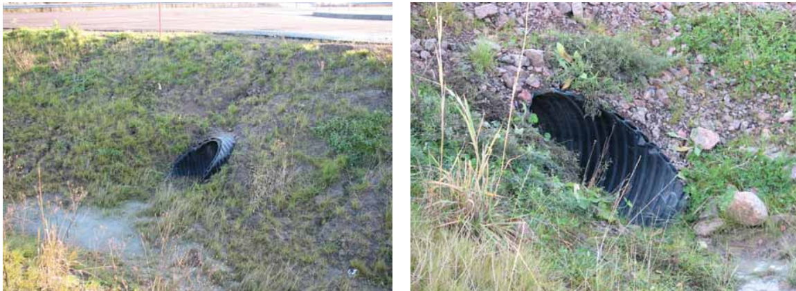
Figure 4.13. Bevelled culvert ends in minor road junctions (Photo, HUT)
