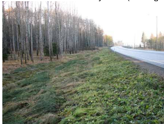
Figure 4.7. Example of a Clear Safety Zone when trees have been removed (Photo, HUT)
