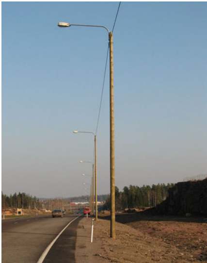
Figure 4.15. Left: Break-away wooden column; glued and laminated. Right: Yielding, energy absorbing steel column (Photo, HUT)
