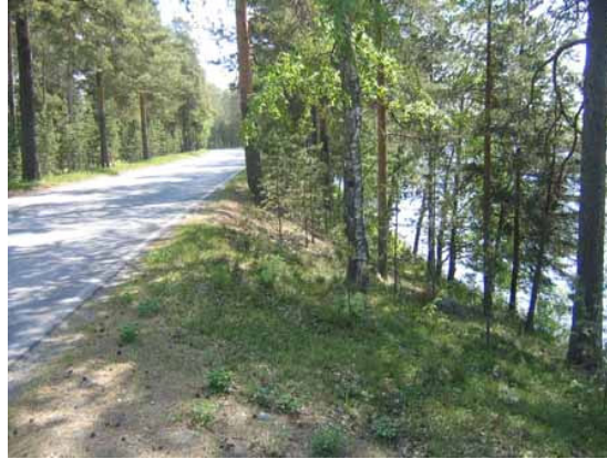
Figure 4.23. There is evident need for better roadside safety because of trees and steep slope. In this road section the only solution for better roadside safety is safety barrier – by choice the guardrail with aesthetical value
