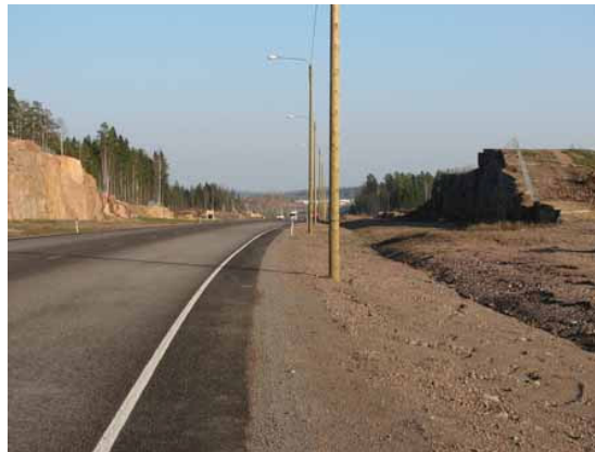
Figure 4.24. Rock face cutting removed from the safety zone (Photo, HUT)
