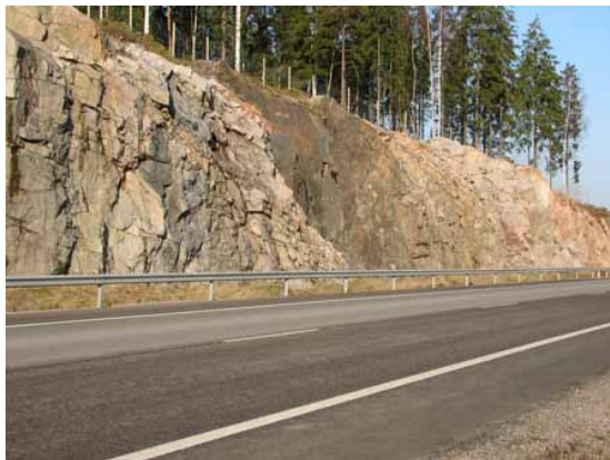
Figure 4.25. Rock face cutting shielded with safety barrier (Photo, HUT)
