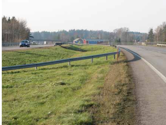
Figure 4.10. Underpass opening on motorway median protected with safety barriers. (Photo, HUT)
