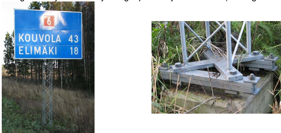
Figure 4.19. Small break-away sign support
