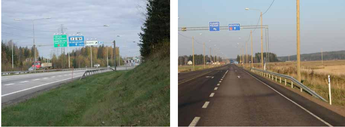
Figure 4.18. Gantry pole shielded with safety barrier, note that the use of unflared, turned down barriers is not recommended (Photo, HUT)
