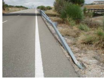
Figure 1.1. Examples of Safety Barrier Terminations, Blunt End, Ramped not Flared End
