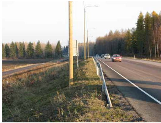
Figure 4.20. Fill slope with a safety barrier, height exceeds 3.0 m.
