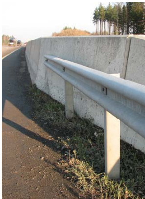
Figure 4.27. Left: good solution of transition structure, the guardrail is overlapped with the concrete barrier and fastened with steel bolt. (Photo, HUT) Right: poor solution of the transition from steel guardrail to the concrete pillar of the bridge parapet. (Photo, VALT)
