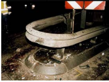
Figure 1.1. Examples of Safety Barrier Terminations, Blunt End, Ramped not Flared End
