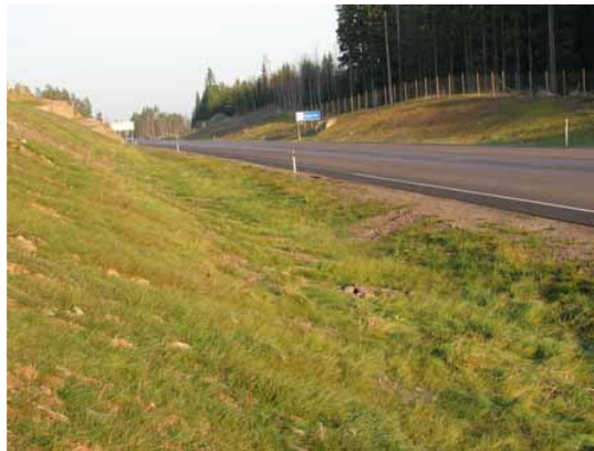
Figure 4.22. Recoverable fill slope; bottom of the ditch is rounded, no hazardous obstacles in fill slope. (Photo, HUT)
