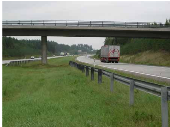
Figure 4.26. Left: too short guardrail, Right: lengthened guardrail (new section with weaker posts). (Photo, HUT)
