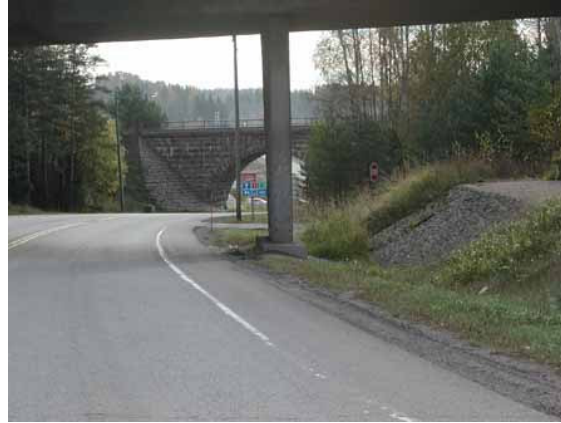
Figure 4.8. Example of hazardous, unshielded bridge pier and bridge abutment
