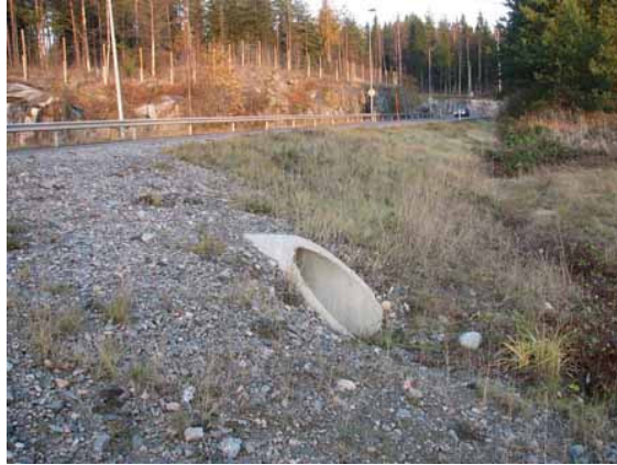
Figure 4.14. Bevelled end of a concrete culvert: safer design than traditional vertical end shape (Photo, HUT)
