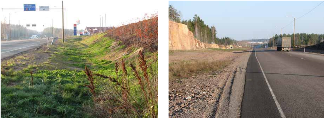
Figure 4.21. Recoverable ditch shapes: 1:4 fore slope, rounded bottom and 1:2 back slope. (Photo, HUT)
