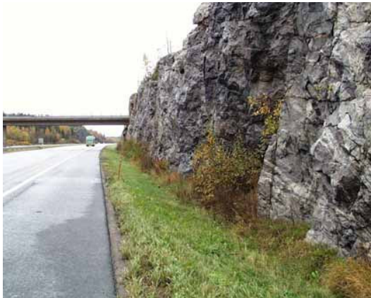
Figure 4.6. Examples of the distributed hazards. Left: unprotected rock cut very close to the carriageway. Right: untested guardrail with concrete posts and too low positioning (Photo, HUT)
