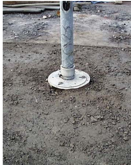
Figure 4.16. Left: old wooden lighting column. Right: old steel lighting column, both are modified to break away at impact.(Photo, HUT)
