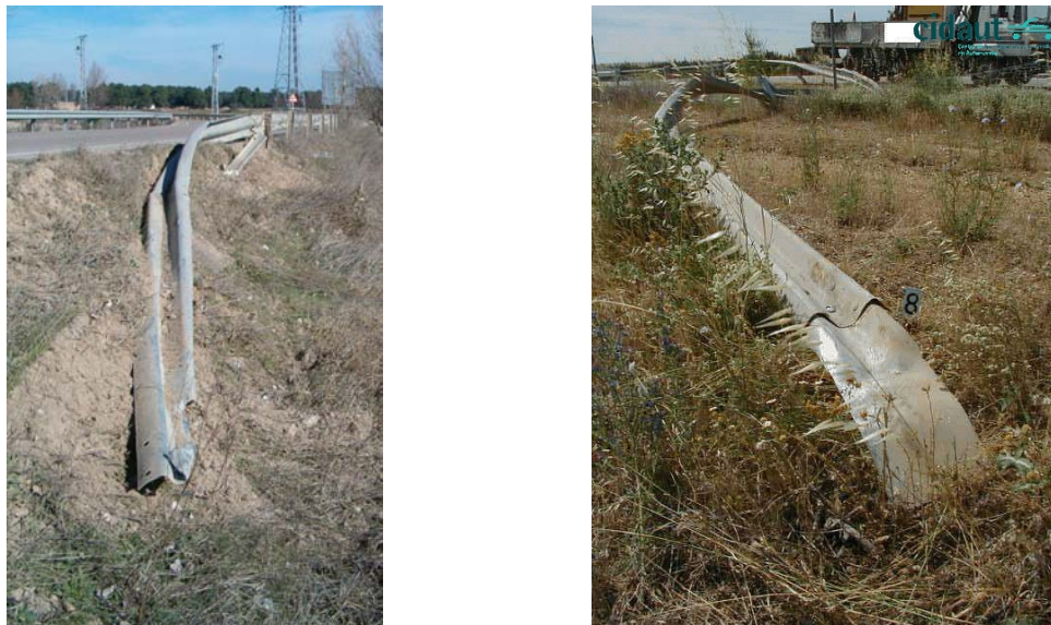
Figure 5.21 Failure in end sections
