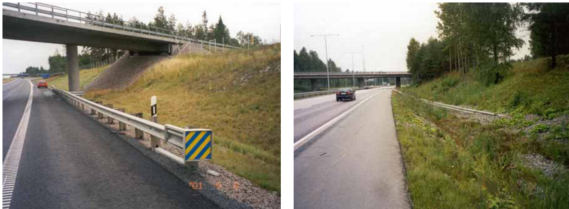
Figure 4.28. Energy absorbing guardrail terminal and flared guardrail terminal (Photo, HUT)
