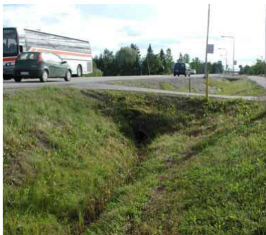
Figure 4.11. Examples of culverts in minor road junctions: traditionally the ends are vertical and the side slopes of the minor roads steep which makes them very hazardous objects in collisions (Photo, HUT)
