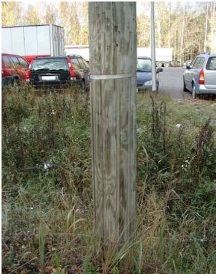
Figure 4.16. Left: old wooden lighting column. Right: old steel lighting column, both are modified to break away at impact.(Photo, HUT)
