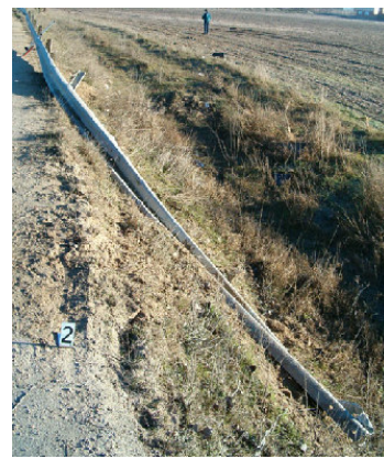
Figure 3.2. Damaged barrier in bend.
