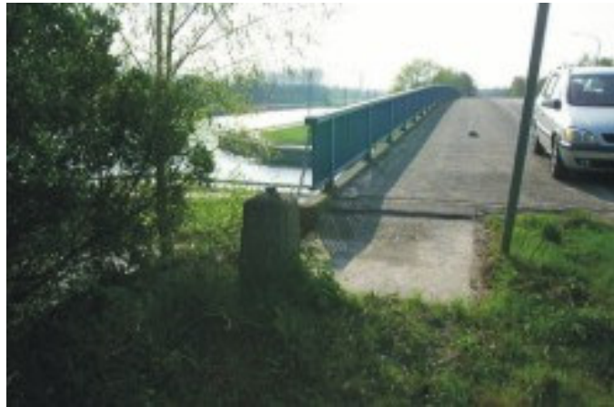
Figure 1.1. Exposed bridge railings.
