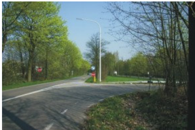
Figure 1.4. Street furniture in a vulnerable position.
