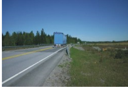
Figure 1.3. Barriers before bridge are too short to stop vehicles from rolling down the steep embankment.
