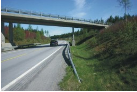
Figure 1.2. The length of the safety barrier would allow a vehicle to go behind the barrier and strike the bridge pillar.
