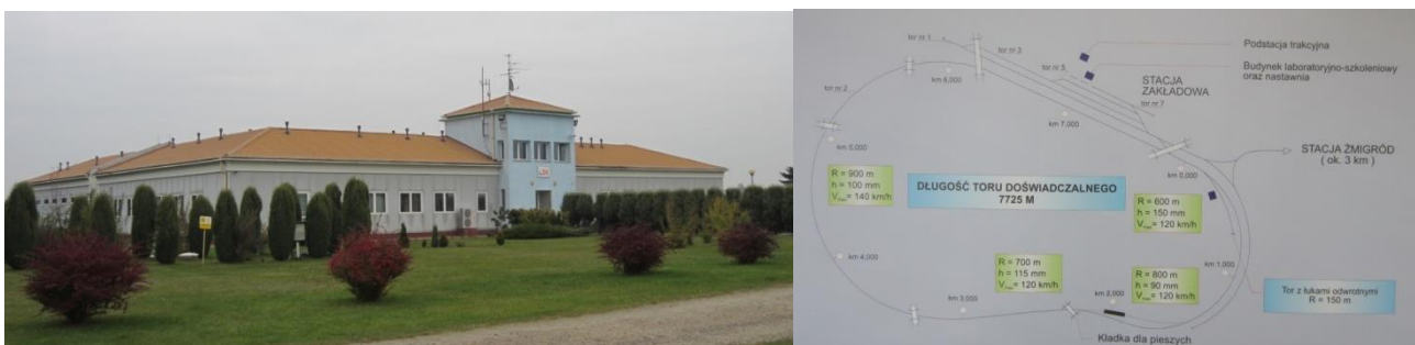
Figure 3: The PROTECTRAIL demonstration was given in Zmigrod in October 2013 at a small station. A photo of the railway station is shown left and the map of the test railway track is shown right.
