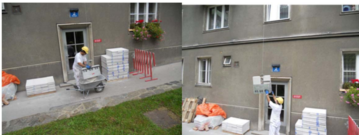
Picture 25: Use of the material hoist
