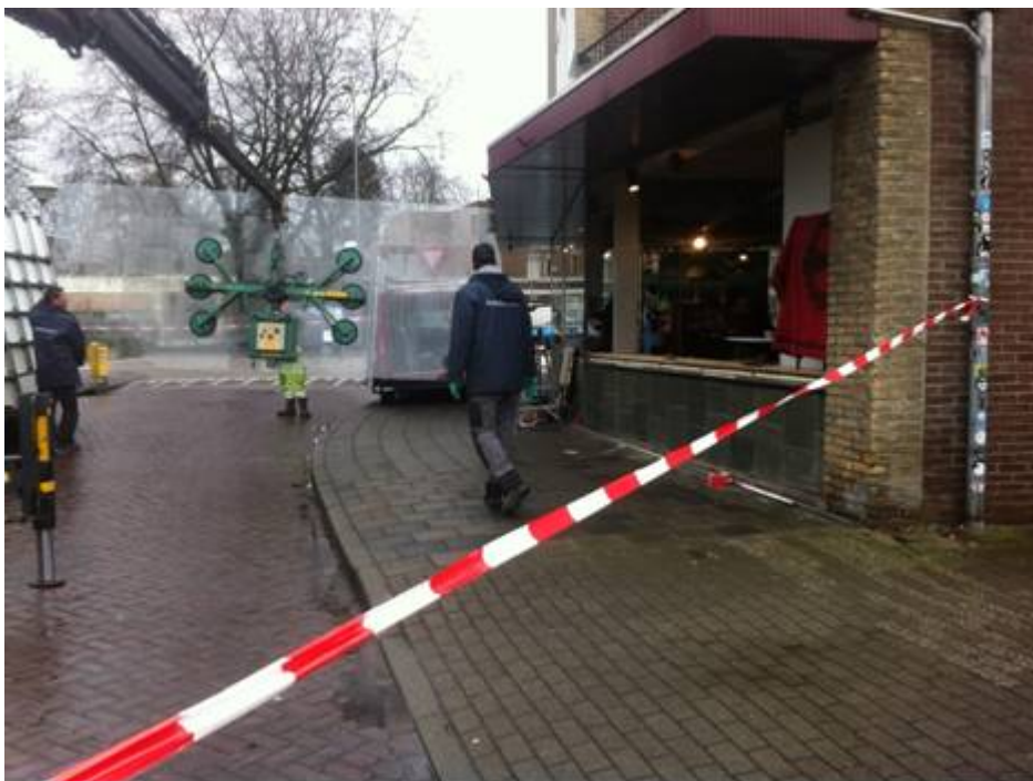
Picture 13: Lifting window panes
