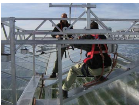
Picture 17: Greenhouse construction and maintenance
