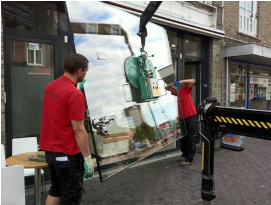
Picture 13: Lifting window panes
