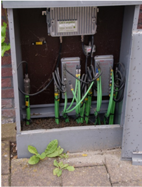
Figure 11: Typical Dutch street cabinet housing the final amplifier (top) and two multi-taps (bottom right) with coaxial drop cables to the connected homes. Source: TNO
