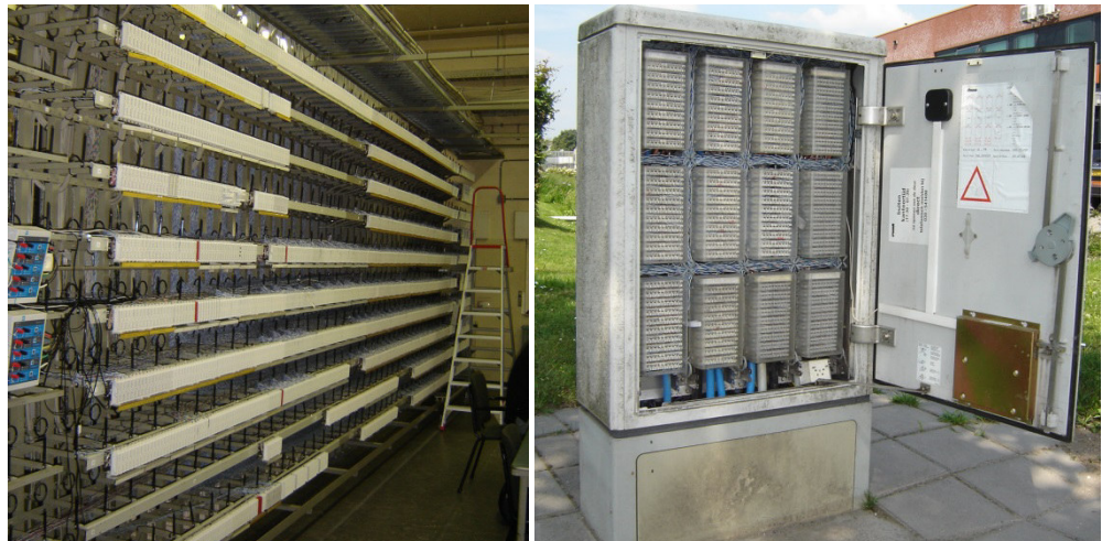
Figure 3: A part of the main distribution frame in a central office (left) and a small cabinet with its sub loop distribution frame inside (right). Source: TNO
