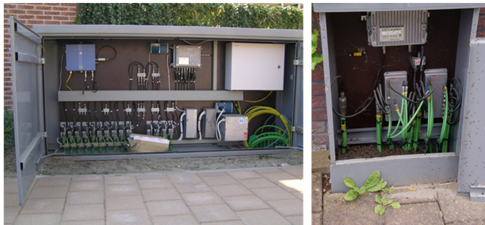
Figure 12: A typical Dutch street cabinet for an optical node (left) and last amplifier (right). Source: TNO
