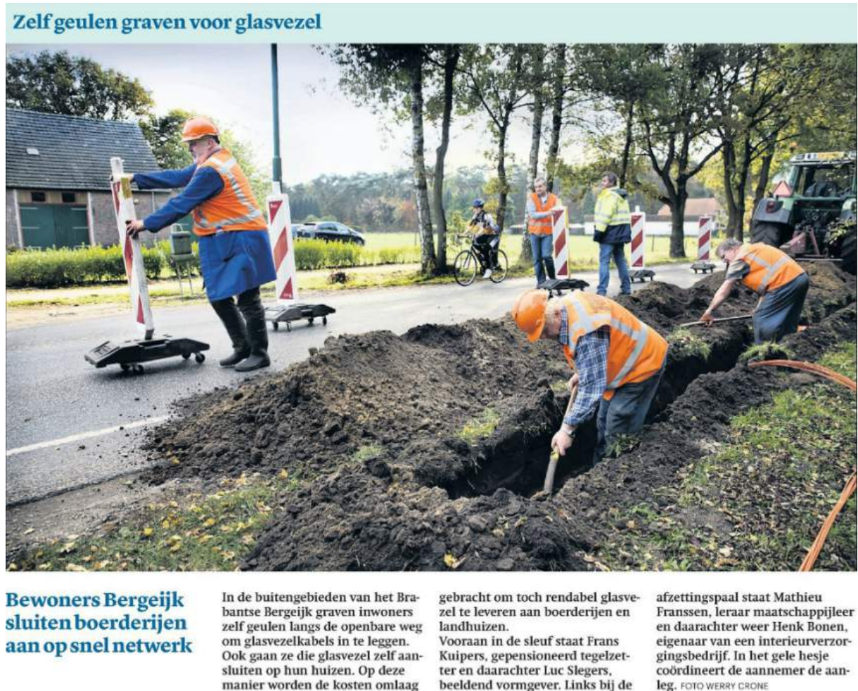
Figure 3.9: Saving costs by digging yourself (source: Trouw 2013).
