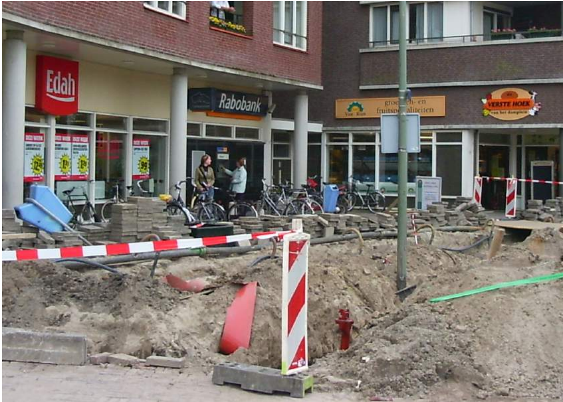
Figure 3.10: Difficult access to stores.
