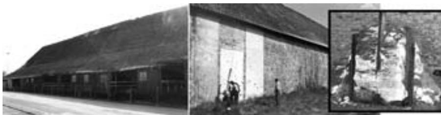
Figure 1: Test site of LRMH at Dieuze. Left: platform for salt transfer, East side; middle: test wall with renders, West side; right storage of salt against wall, inside.
