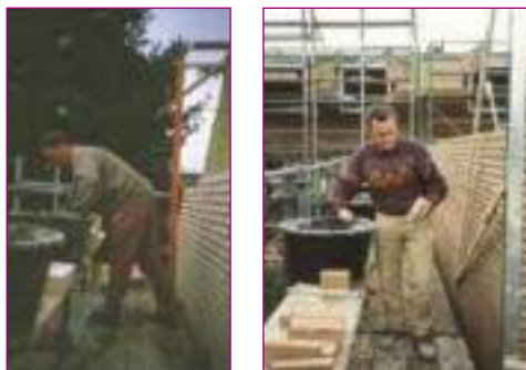
Figure 15. Raised bricklaying
